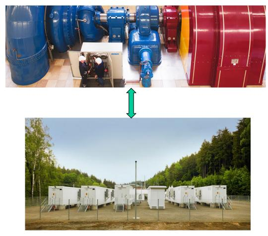
Hybrid pumped-storage+Li-ion batteries ESS in Pfreimd hydropower system, Germany. Taken from <u>https://www.engie-deutschland.de/</u> and <u>https://blog-</u> tractebel.lahmeyer.de/
