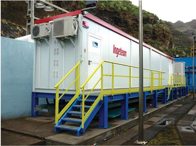
4-MW/5-s **supercapacitor** ESS installed in La Palma island, Spain. Taken from P. Fontela et al., Canary Islands Benefit from Enhanced Grids, T&D World, 2015.
