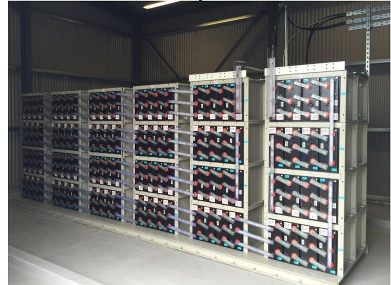
**Hybrid flywheel+lead-acid batteries ESS** in Rhode, Ireland. Taken from <https://schwungrad-energie.com/>
