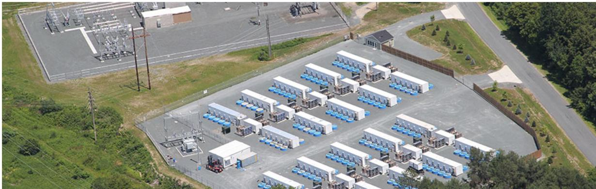
20 MW/15-min. **flywheel** ESS installed in Stephentown Supercapacitor installed in Stephentown, NY, USA. Taken from <https://beaconpower.com/>.
