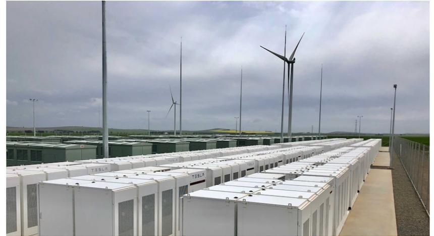
150-MW/189-MWh **battery** ESS installed in Hornsdale, Australia. Taken from S. Tomevska, Tesla battery in South Australia expanded by 50 per cent energy minister lauds benefits, ABC News, 2020.
