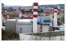
Figure 4. District heating CHP plant with 5500 m<sup>3</sup> water heat storage.
