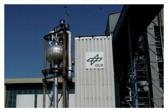
Figure 17: Latent storage system with 700 kW power, 1h storage capacity, Source: DLR.
