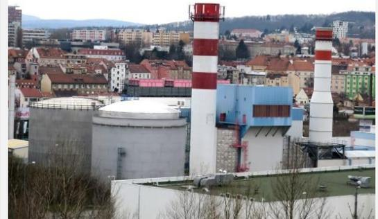
Figure 4. District heating CHP plant with 5500 m<sup>3</sup> water heat storage.
